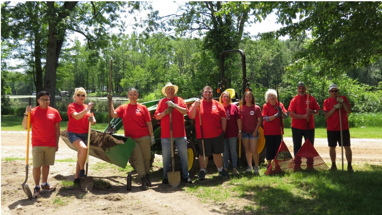
Volunteers help construct accessibility improvements with funding assistance from an AARP grant.
