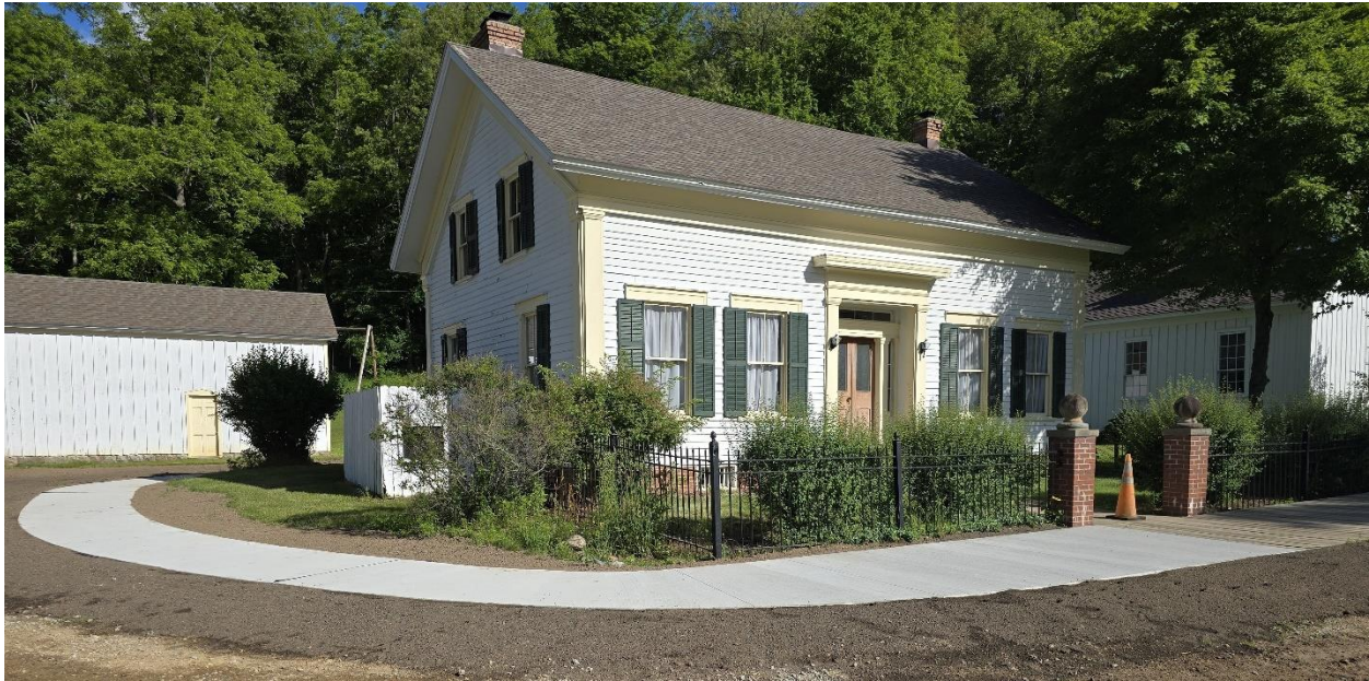
New sidewalk provides improved access to the Sixberry House in Historic Charlton Park Village
