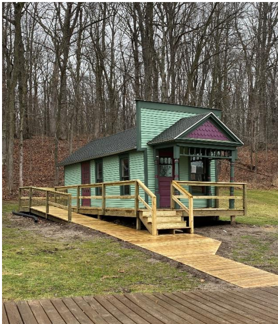
New accessible ramp to the barber's shop
