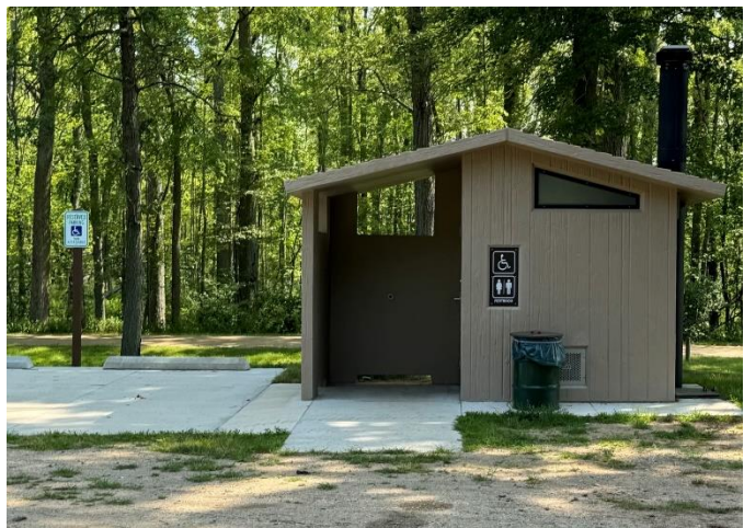
An accessible vault toilet at the boat launch
